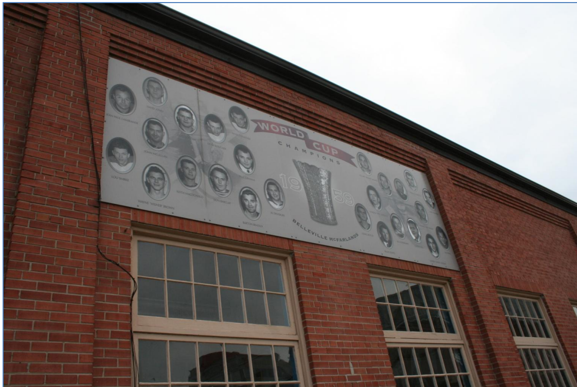
Plate 22: Commemorative signage located on the Memorial Arena.
