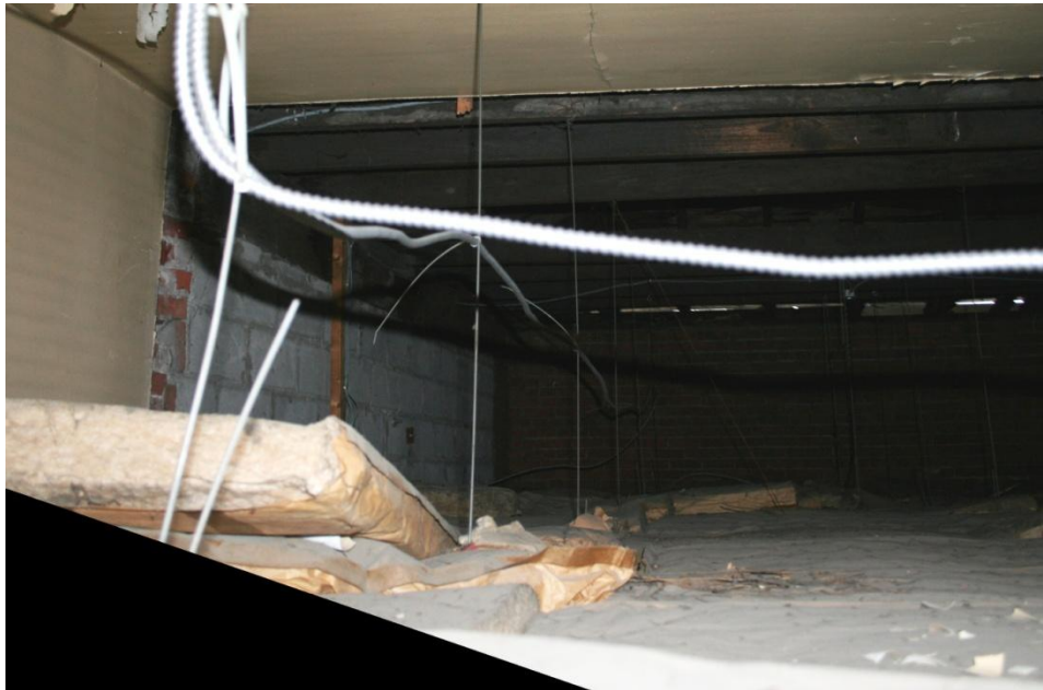
Plate 54: Above the false ceiling in the Weigh Scale Building. Note the beam structure and where the wall and roof coverings end.
