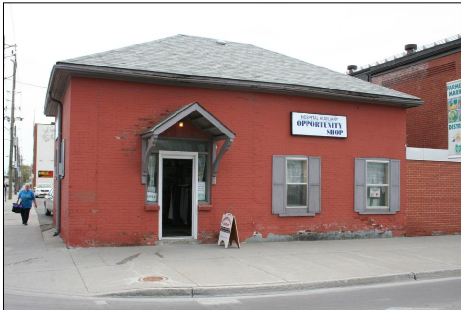
Plate 47: The Weigh Scale Building.
