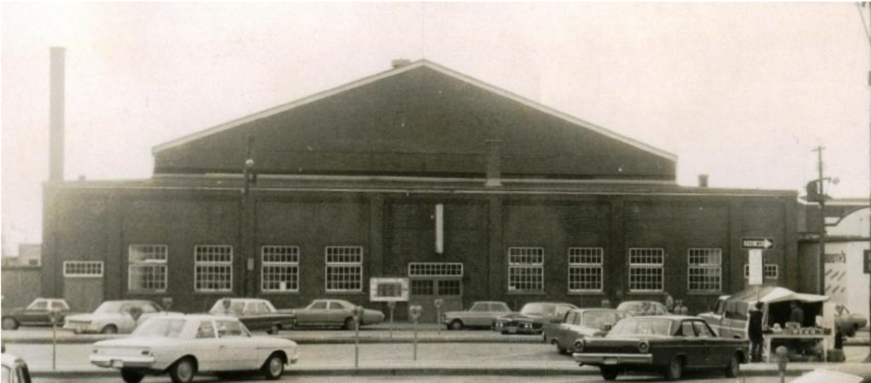
Plate 32: Memorial Arena (c. 1970) showing the original door and window pattern. Source: Community Archives of Belleville and Hastings County, Mika Collection.
