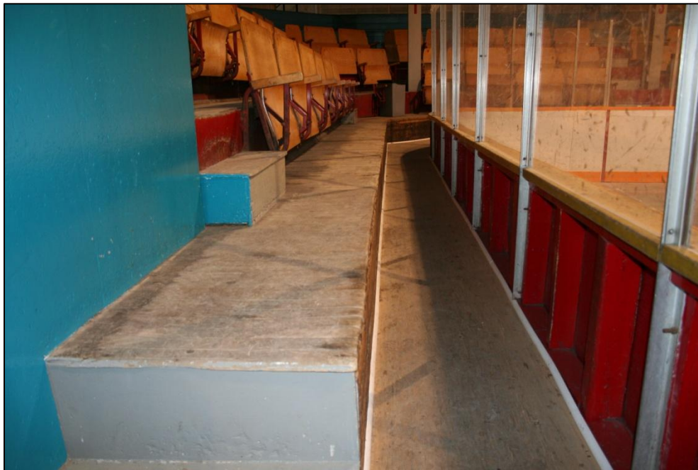
Plate 37: The original seating risers at the north end of the Memorial Arena. The wooden seats were later additions.
