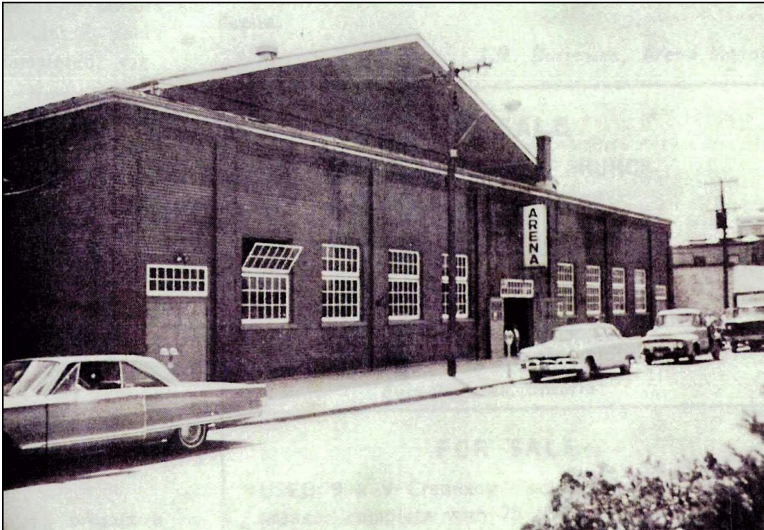
Plate 31: Memorial Arena c 1970. Note the opening windows and the original structure of the main entrance. Source: Burrowes, 1970.
