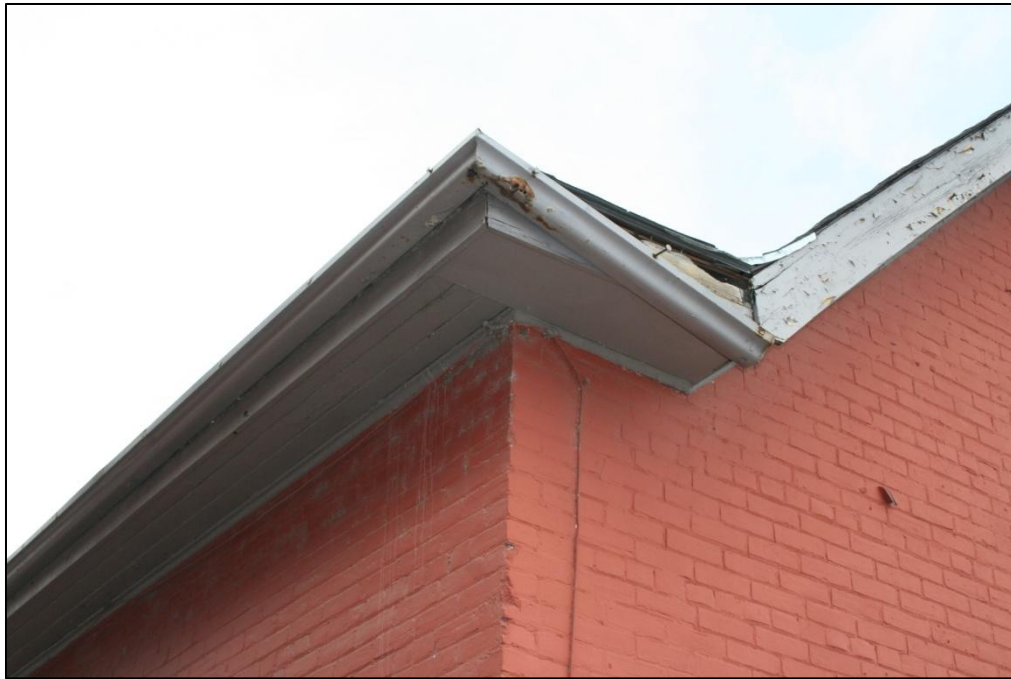
Plate 52: Soffit and Fascia detail on the Weigh Scale Building.
