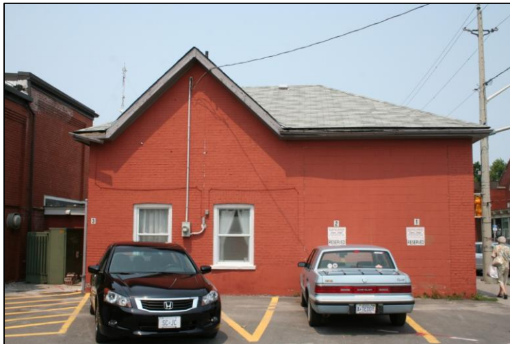
Plate 51: Rear of the Weigh Scale Building.
