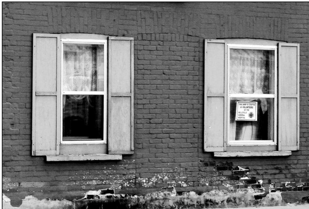
Plate 53: The Weigh Scale Building with its bricked-in door.
