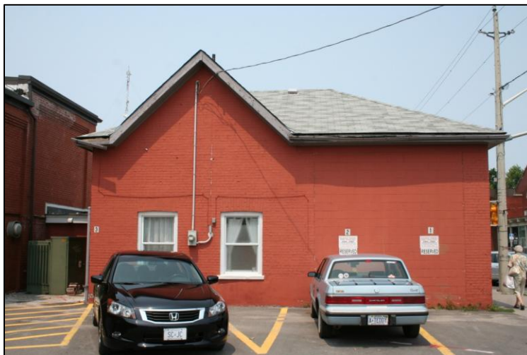
Plate 51: Rear of the Weigh Scale Building.
