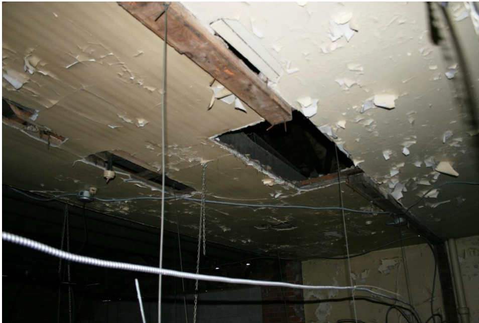
Plate 55: Above the false ceiling in the Weigh Scale Building. Note the use of lath-and-plaster.
