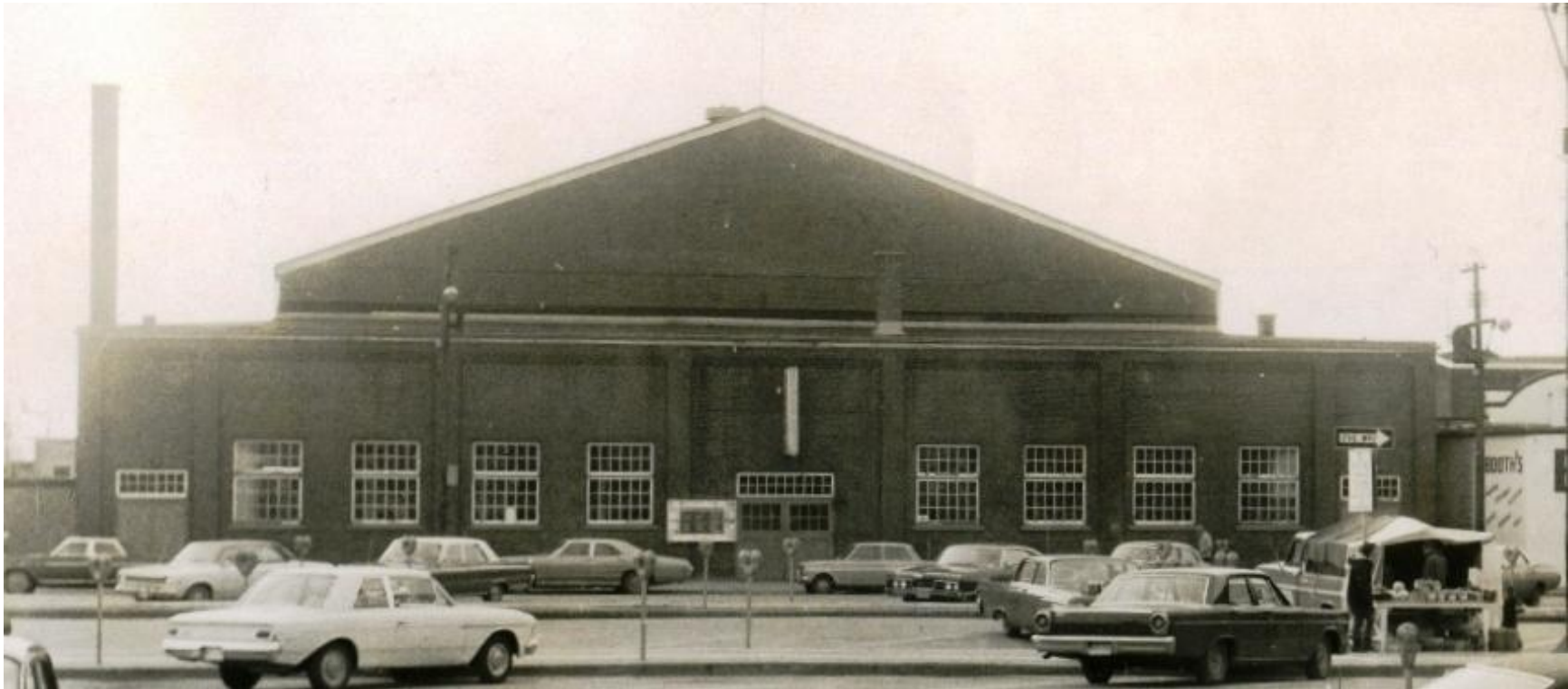
Plate 32: Memorial Arena (c. 1970) showing the original door and window pattern. Source: Community Archives of Belleville and Hastings County, Mika Collection.
