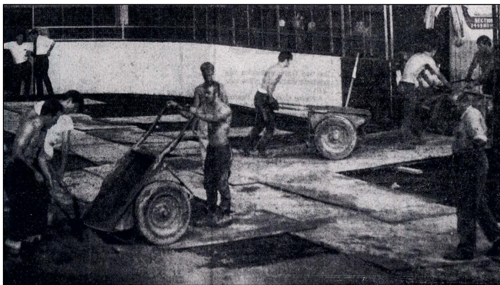
Plate 45: New concrete floor being poured into the Arena. Source: Unknown, 1967.
