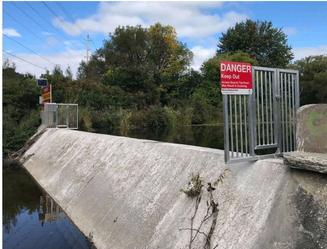
Picture taken looking north across spillway.
