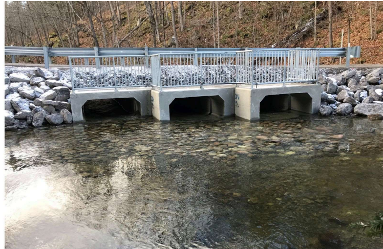
Completed construction, undertaking fall drawdown. Taken from the upstream left bank.
