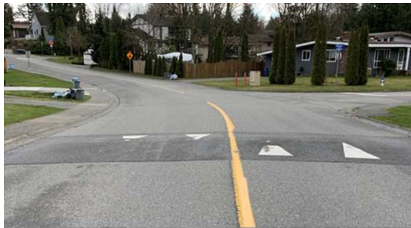
Figure 4-63: Example of a Speed Bump, Source: City of Abbotsford
