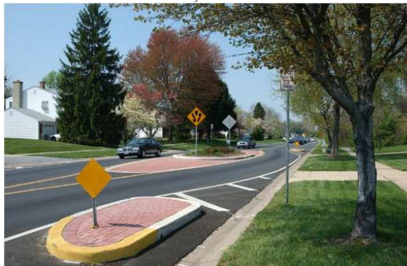
Figure 4-64: Chicane on a Residential Road Source: NACTO (National Association of City Transportation Officials)
