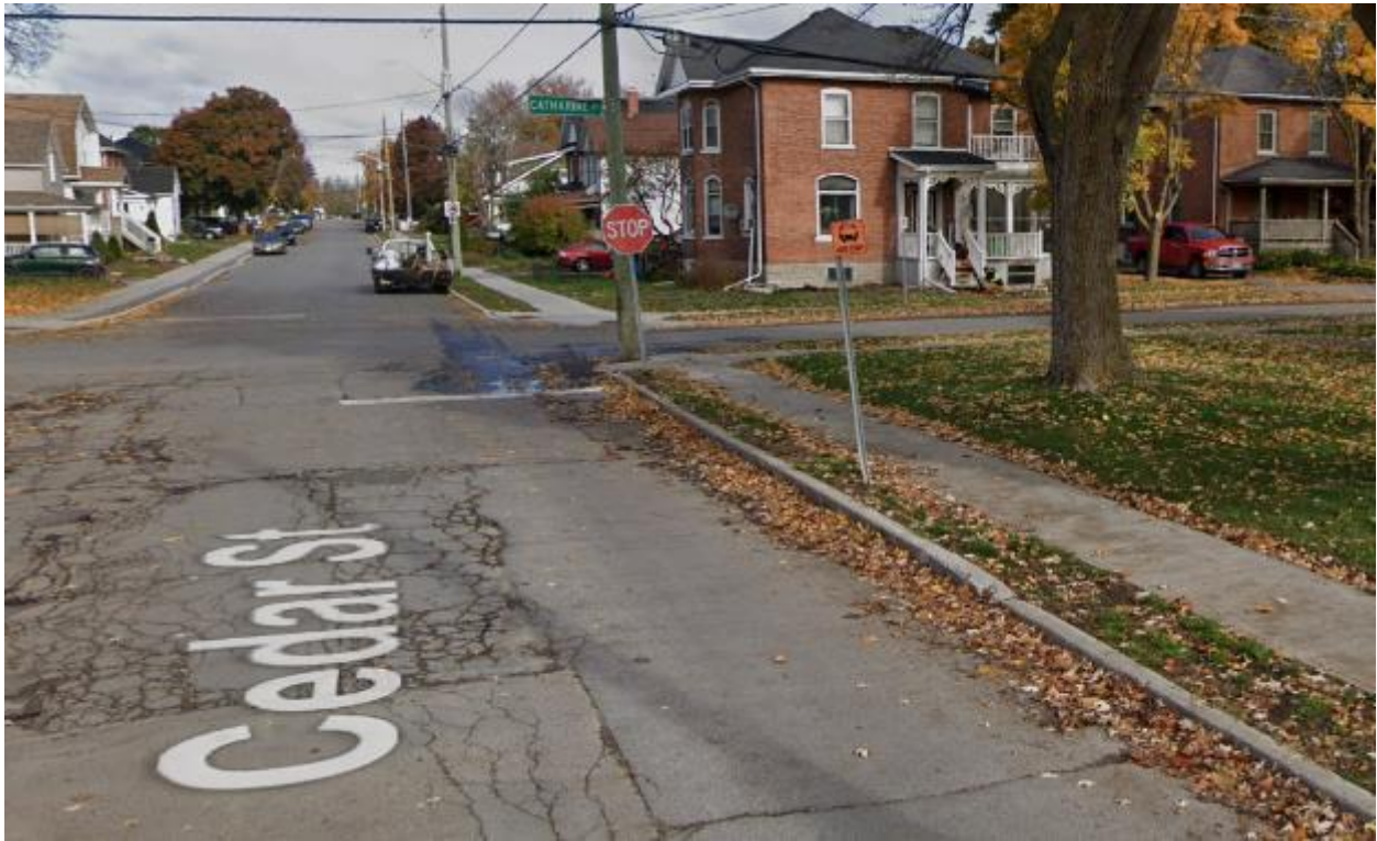
Figure 61: Belleville Transit Bus Stop on Cedar Street at Catherine Street. This is a near-side stop on a neighbourhood street with no pad or shelter. Insufficient space between stop sign and intersection.
