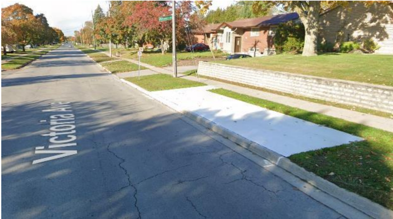
Figure 65: Belleville Transit Bus Stop on Victoria Avenue at Parrott Drive. This is a far-side stop on a neighbourhood road with an appropriately sized pad
