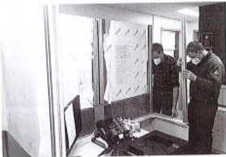
Installed Pull-Across Barriers
