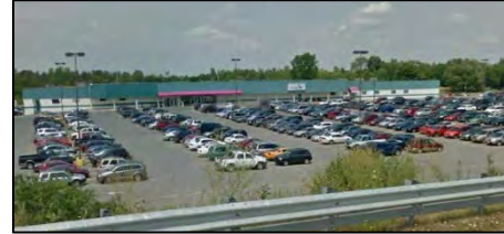
Stream Call Centre (89,000 sq.ft. G.F.A.), site of former retail centre.
