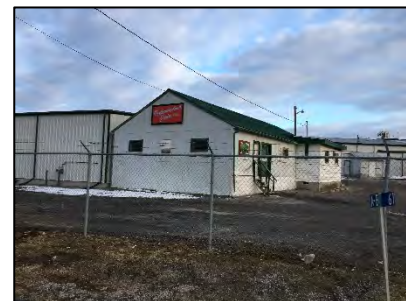
Northumberland Grain Inc., 61 Tank Farm Road.
